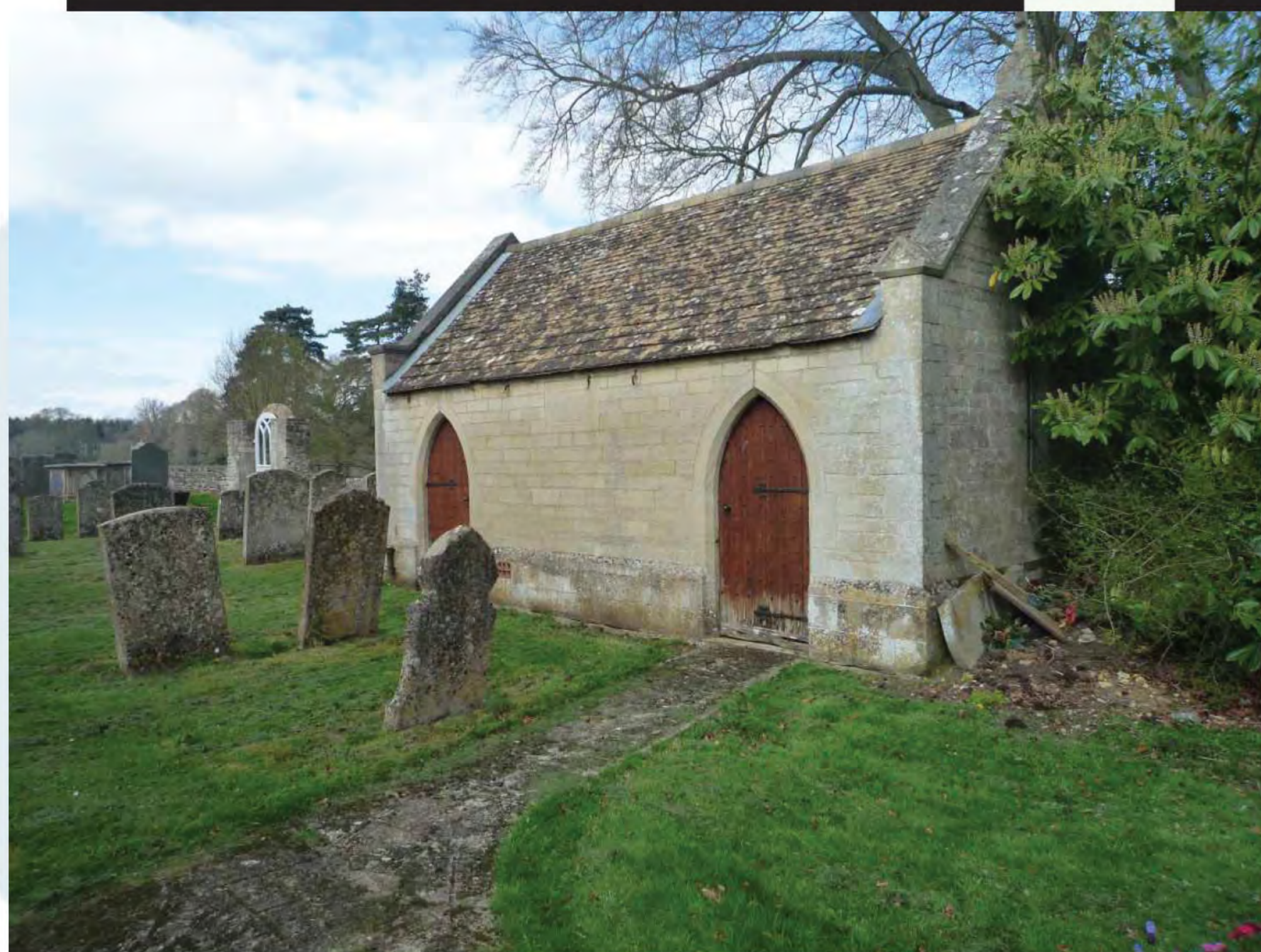
Exton Church Toilet and Kitchenette
